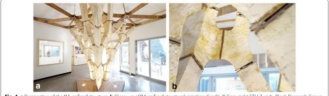
Fig. 4 a Perspective of the "MycoTree" structure. b Close-up of "MycoTree" structure's jointing. Credit: © Copyright ETH Zurich, Block Research Group. / Photographs by Carlina Teteris [13]
